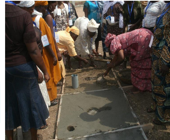
Training on slab construction for women in Osun State, Nigeria
